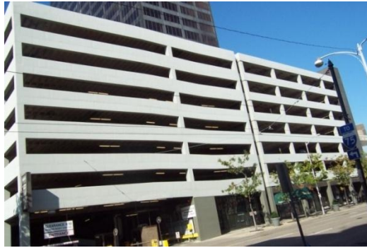
Figure 11. AMPCO Parking Garage, Dayton Ohio
