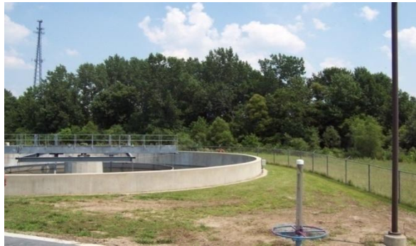
Figure 13. Green County Waste Water Treatment Facility Processing Tank
